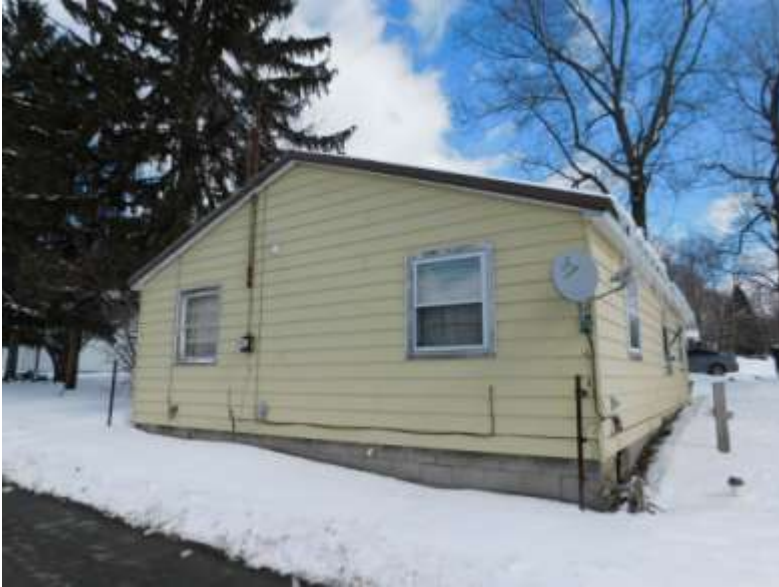
Rear View of Accessory Single Family Unit Building
