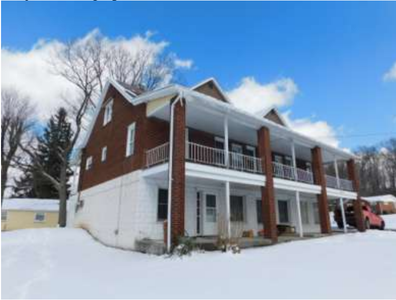
Left Side & Front Views of Apartment Building
