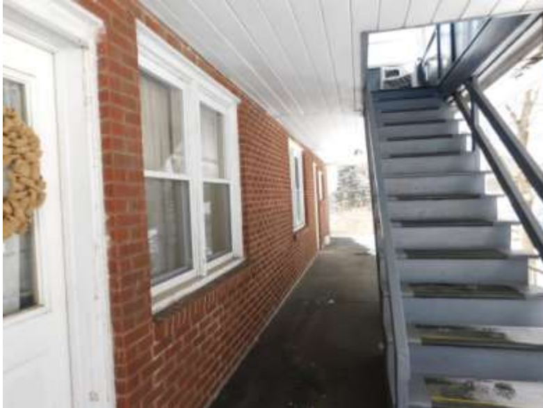
Stair Access to Third Floor
